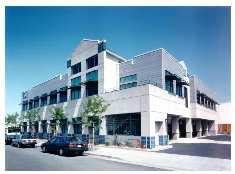
MFT provided structural engineering for this CalSport Partnership office building. The 17,000 sf mixed-use building was comprised of two stories of structural steel and wood frame construction. Physical therapy rooms and additional sports medicine facilities were located on the second floor, with retail shops on the ground floor.
