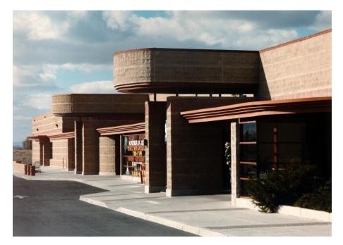
MFT provided structural design services for the 23,000 sf expansion and remodel of the Fallon Naval Air Station Commissary. The structural system consists of steel framed roof system supported by reinforced masonry bearing and shear walls on a slab on grade foundation.
